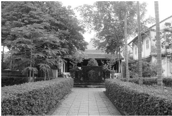
Fig. 2: Outer screen in front of the main house
