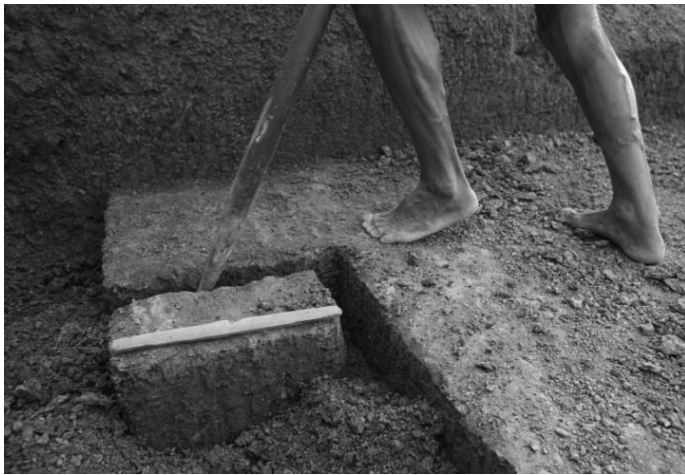
Fig. 5: The worker uses a special tool (Thó) to mine laterite
