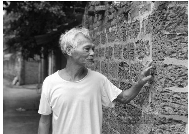
Fig. 10: Ancient laterite brick wall, linked by clay
