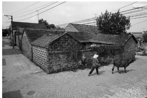
Fig. 12: Village roads and houses built from laterite brick in Duong Lam ancient village
