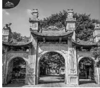
Fig. 8. Three-entrance gate made of stone
