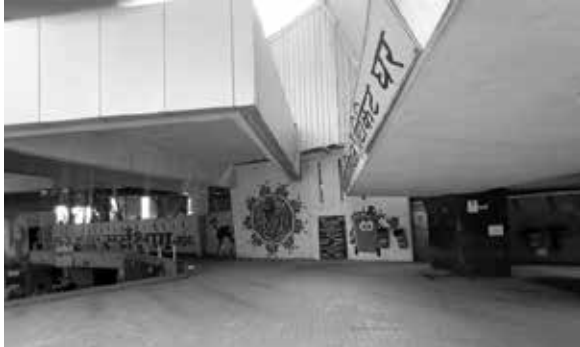
Fig. 6. East side entrance of Ghansoli suburban train station, Navi Mumbai. Exterior paints 2021
